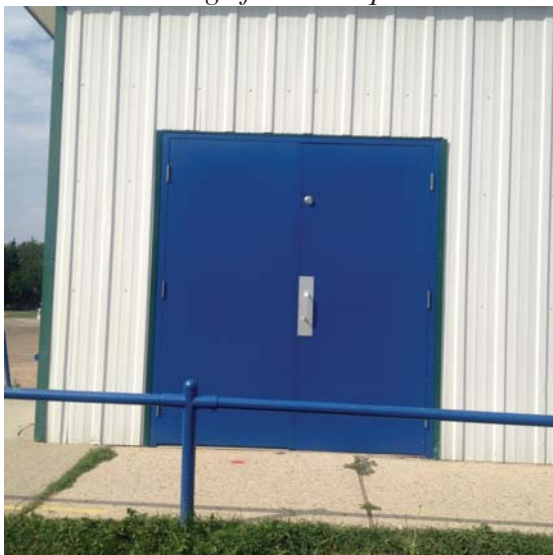
Photo 20. Storage for barbeques.
