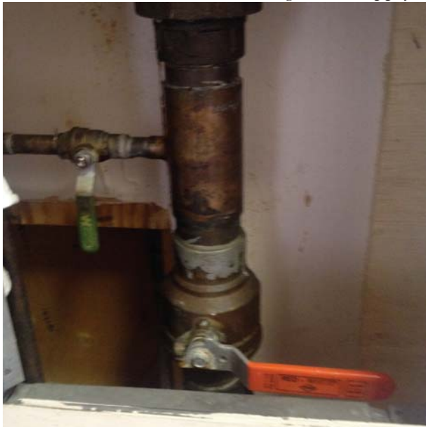
Photo 22. Valves controlling water supply to rink hose.
