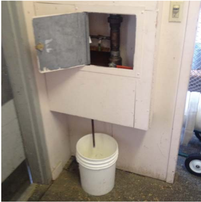
Photo 22. Valves controlling water supply to rink hose.
