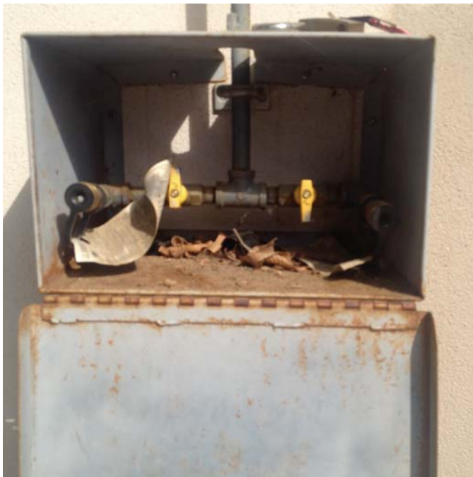
Photo 22. Gas outlet box opened.
